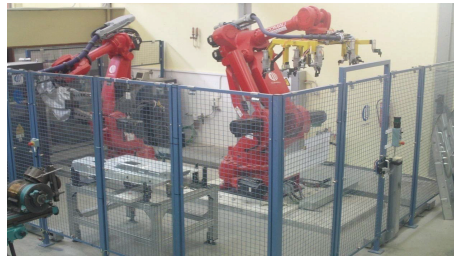
Figure 4: Actual assembly cell.
