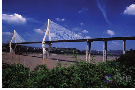
Figure 5: A picture of the Chongqing MaSangXi Grand Bridge.
