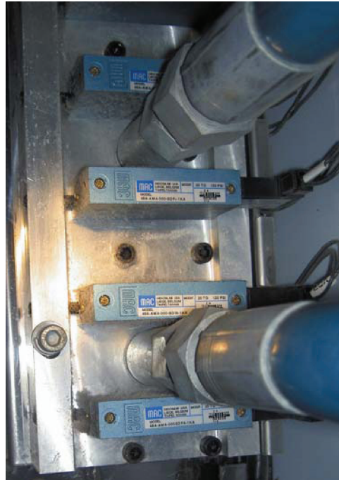
Figure 7: Solenoid valves.
