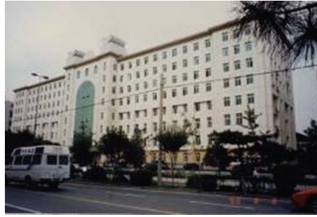
Figure 17: The photo of story-increased building.
