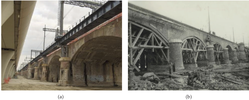
Figure 1: (a) Longitudinal view of the multi-span masonry arch bridge as appears today and (b) view of a construction phase, presumably dated around 1852.
