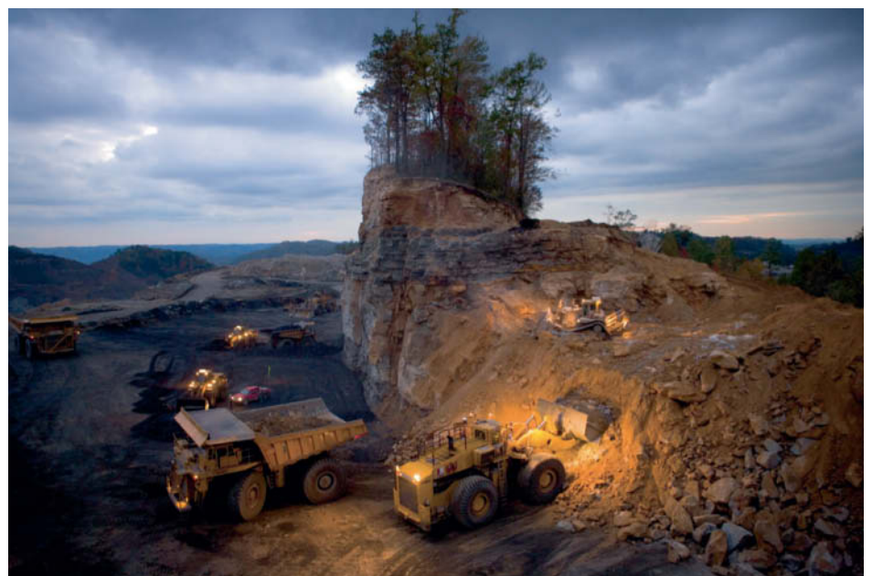
The Last Stand Kayford Mountains, West Virginia, USA Blasting spoil being removed by machine. Modern mining operations work around the clock and at amazing speed. This lonely stand of trees disappeared in less than a day.
